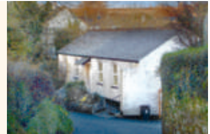
£3,500 for urgent repairs brought Kingston Reading Room, Devon, back into the heart of the community.
