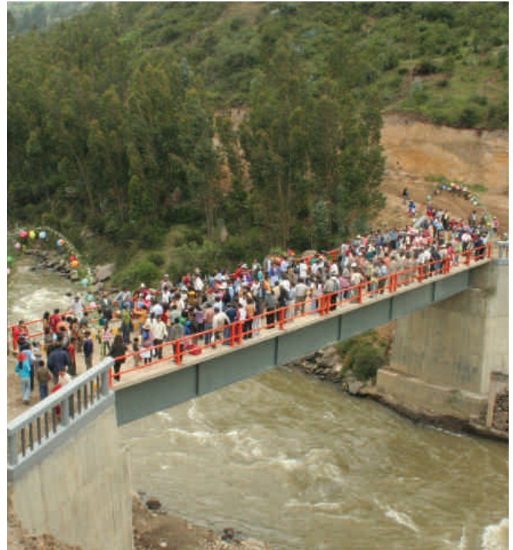
COMMUNITY MEMBERS INAUGURATE A NEW BRIDGE SPANNING THE SANTA RIVER.
