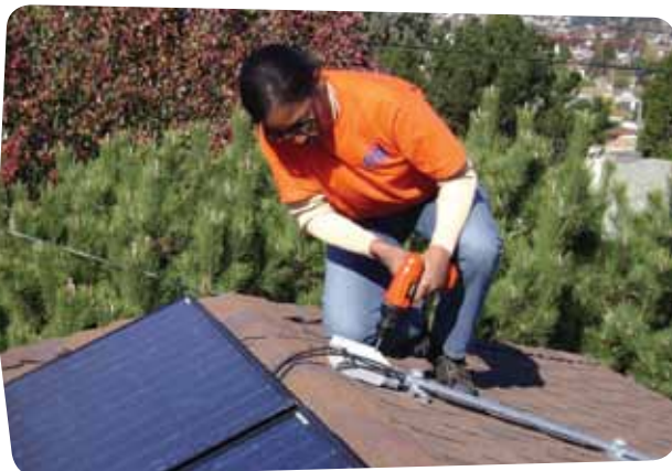
A Solar Richmond graduate installs panels on a neighborhood house
