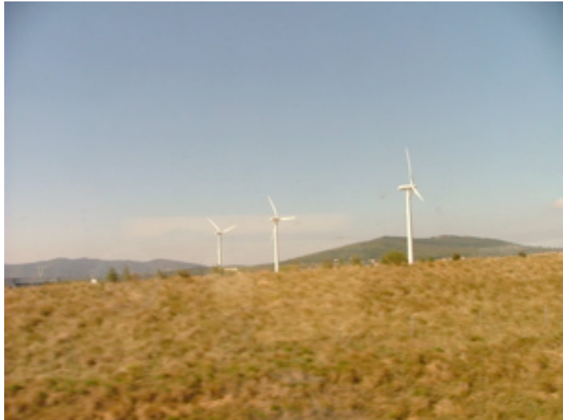
Wind Farm in France near TGV Rail Lines. Photo courtesy of Darcy Hitchcock.
