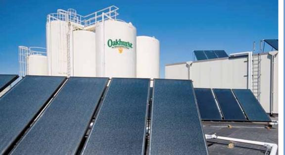
Installation of approximately 2,500 square feet of solar panels on the roof of its Portland headquarters helps reduce the consumption of heating oil by more than 5,000 gallons per year.
