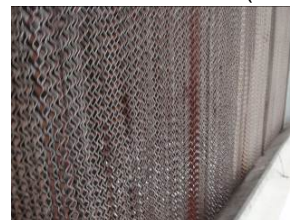
Figure 1. Water Curtain Cooling System
